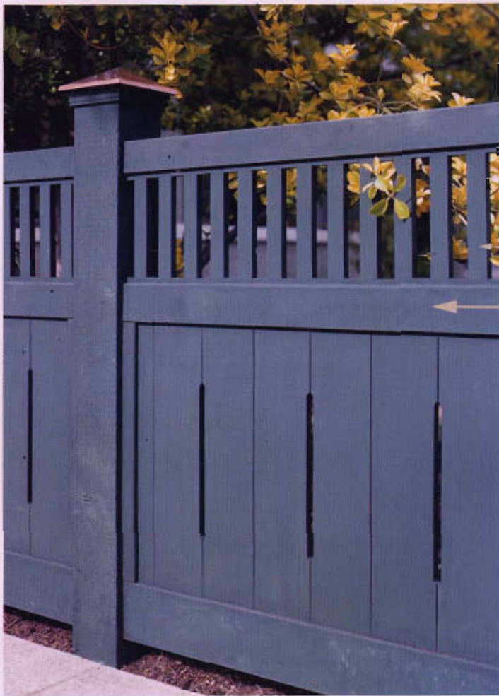
Board fences may be common, but they don't all need to look the same. The good-neighbor fence above alternates boards, making it equally good-looking on both sides. Fast-growing trees, 5 feet apart, offer extra privacy only two years after being planted. At right, fluted joints and a "piano-key" top section add a touch of openness to a green-painted Craftsman fence. Below, rustic grapestakes fill in between more formal brick pilasters.
