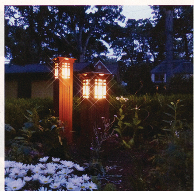
A pair of lighted columns located in the garden are similar in design and construction to the corner column located on the deck, but vary slightly in size.
