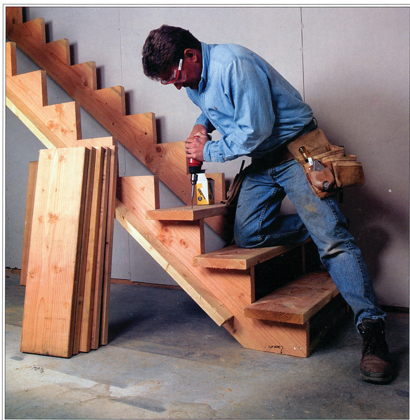
Cutting out Basic Stairs
