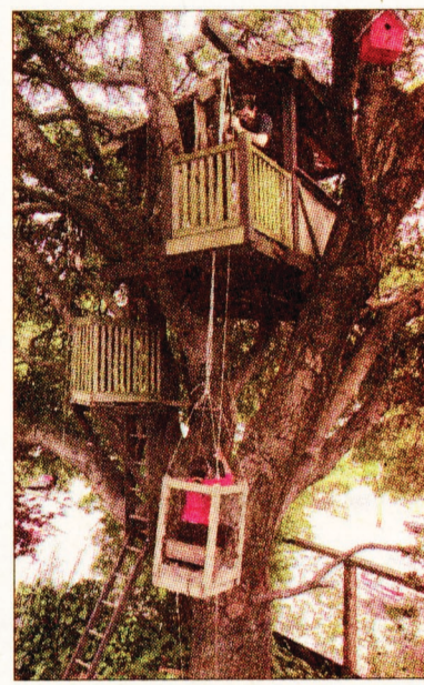
Charlie Prowell built a treehouse in an oak in Sebastopol. The house includes a lift built with pulleys and counterweights.
