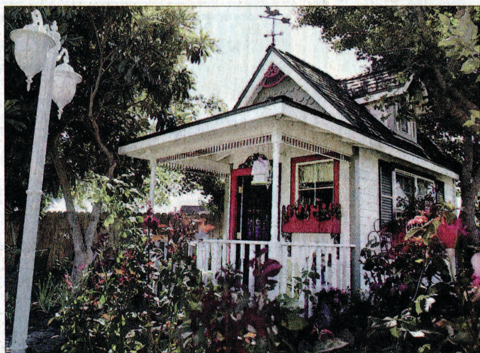
A Victorian-style hideaway built in Anita Rackerby's backyard has low-voltage electricity and a loft. The hideaway is decorated with discounted items found in stores and at flea markets.
